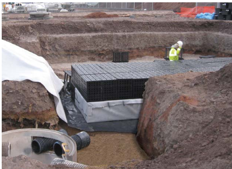
ACO StormTank attenuation system with ACO Q-Brake Vortex flow control
