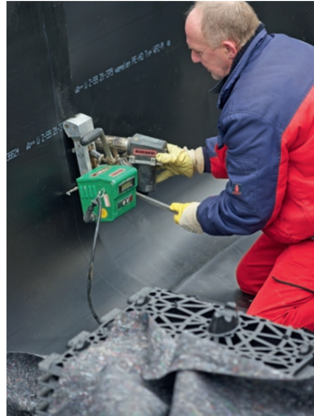
The sealing membrane is then welded
