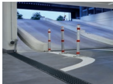
ACO PowerDrain heavy-duty channel with integrated damping
