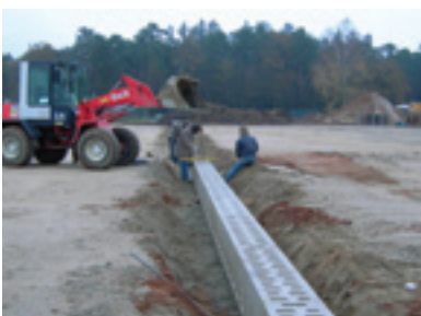
ACO DRAIN® Monoblock RD300 – hitra in enostavna vgradnja
