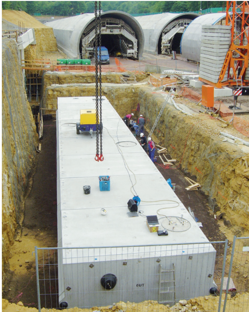
ACO large containers as emergency tanks with fire-extinguisher containers at the Stafelter tunnel
