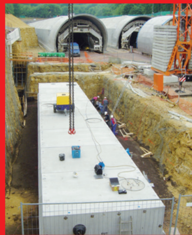
ACO large containers as emergency tanks
