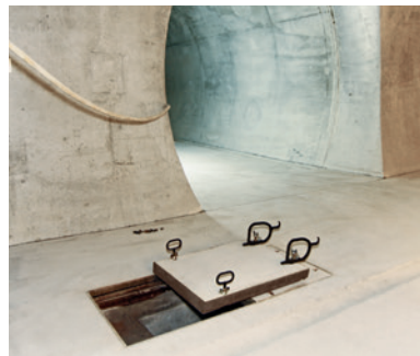
Open shaft manhole cover
