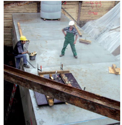
Installation example: 100,000 l fire extinguishing water tank, Mainz University, Germany
