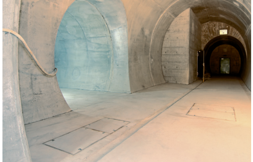
ACO Secant manhole covers used as inspection covers in Wattkopf tunnel
