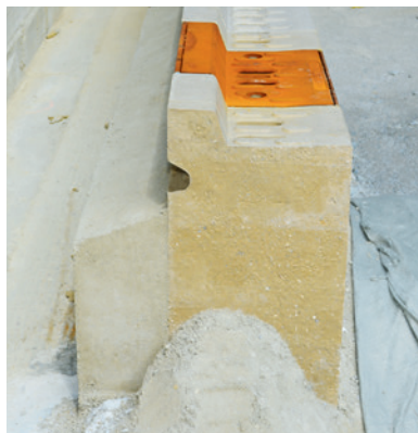
Tunnel channel and foundations parted off on the roadside with a back support on one side
