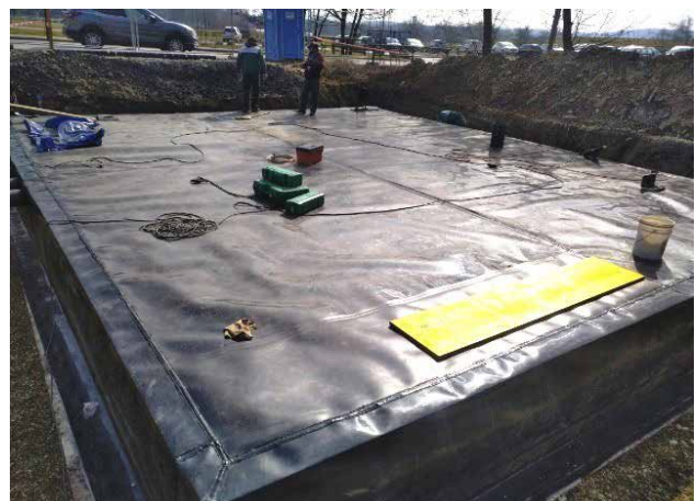
Precise tailoring of the geomembrane around the perimeter of the retention with thoughtful switches with combination of automatic and extrusion welding for 100% waterproofing.
