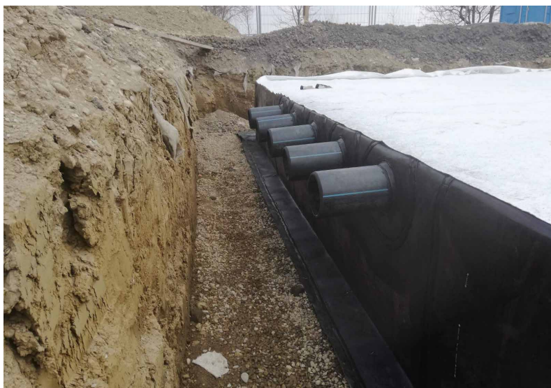
Preparation of 100% waterproof pipe breakthrough for waterproof connections to the pipe. The pipes have to be made of PEHD and smooth from outside.
