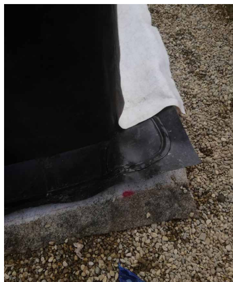
Detail of the longitudinal weld of horizontal geo membrane laid on the floor and side geo membrane of the retainer.
