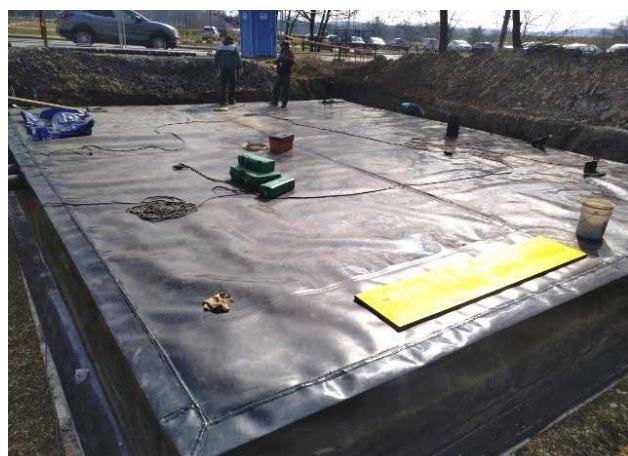
Precise tailoring of the geomembrane around the perimeter of the retention with thoughtful switches with combination of automatic and extrusion welding for 100% waterproofing.
