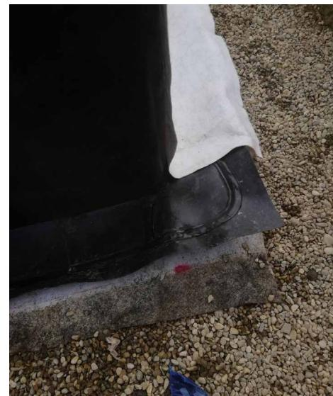
Detail of the longitudinal weld of horizontal geo membrane laid on the floor and side geo membrane of the retainer.
