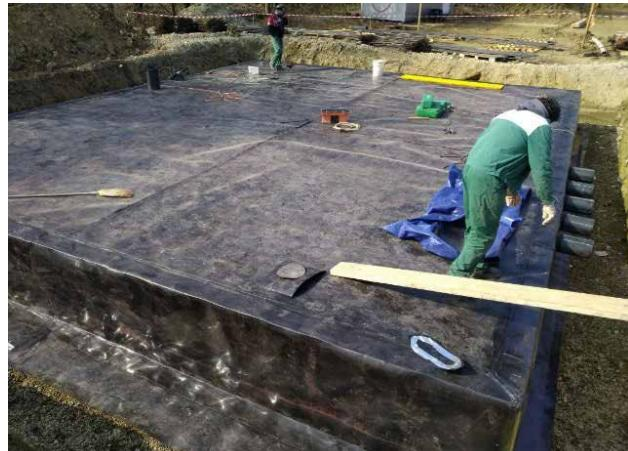
A retention with dimensions 10.8 x 9.0 x 0.91 m and volume of 85 m<sup>3</sup>, is installed under the customers car parking area. The thickness of the cover (backfill soil and the upper road structure of the parking area) is 1.4 m.
