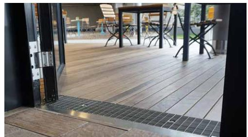
The installation of the ACO Profiline drainage channels next to the panoramic door enables the transition from the building to the wooden terrace without architectural barriers.
