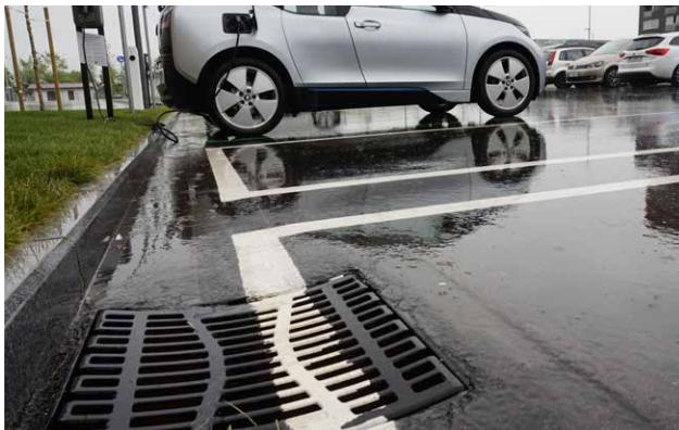
**Multitop inlet grating** with inserted bucket for coarse dirt and geometry of slots, which is safe for pedestrians and cyclists.
